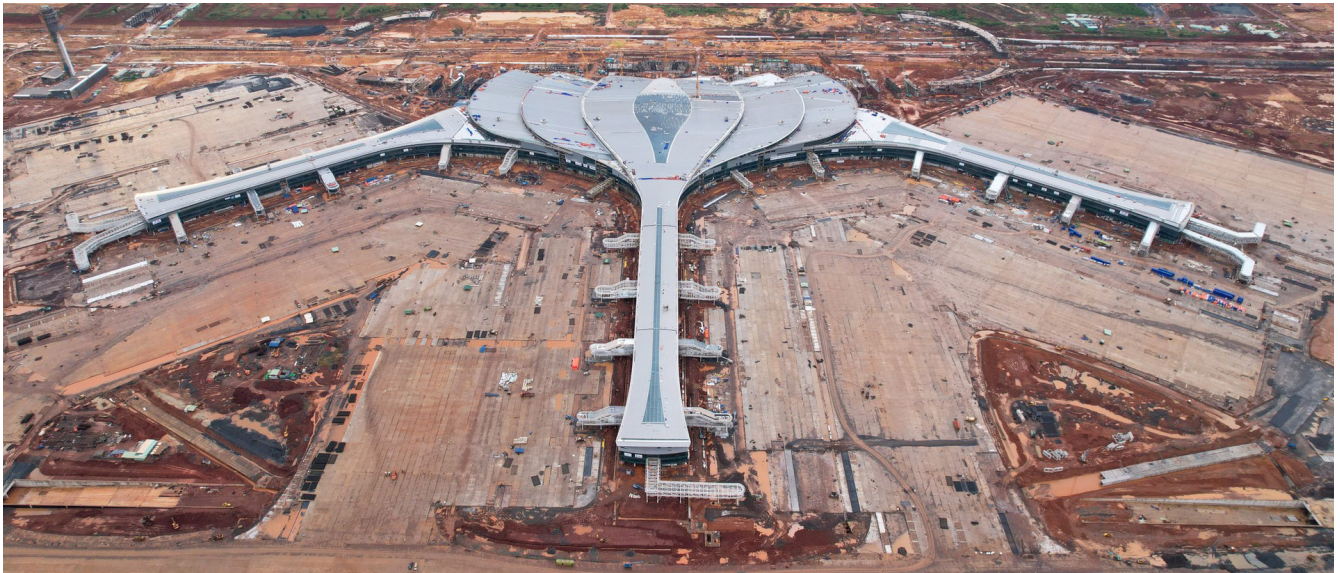
Aerial view of Long Thanh International Airport as of December, 2025. Photo: Wikimedia Commons 18
